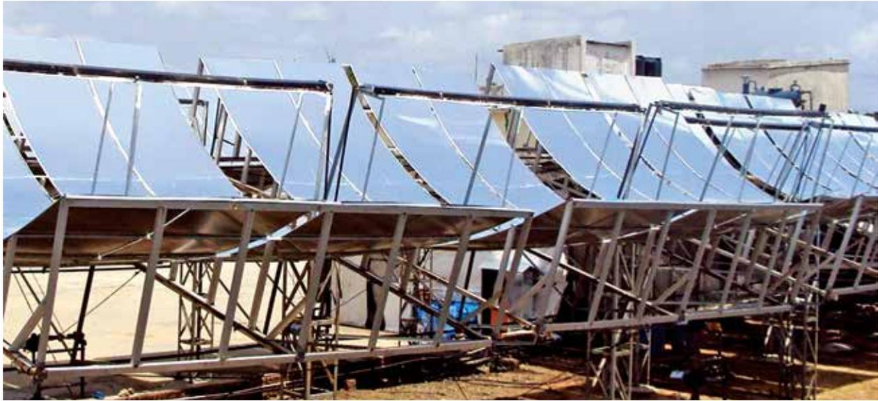
The SharperSun Space Frame was specially designed to reduce the assembly time on the ground and reduces auxiliary power consumption, besides being durable and corrosion-resistant. The SharperSun team is now working on an innovative single-axis tracking system that significantly reduces auxiliary power consumption required for tracking.
